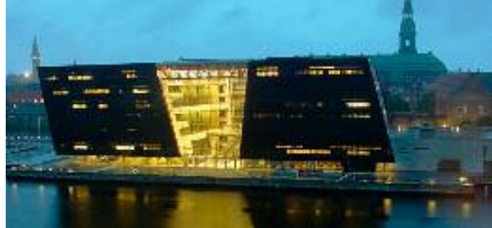
Black Diamond building, Royal Library, Copenhagen
